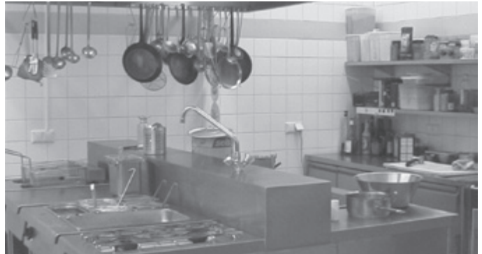
Filter monitoring in kitchens
