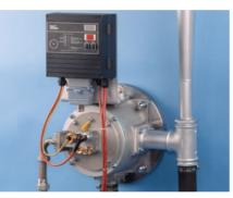
BCU on radiant tube burner
